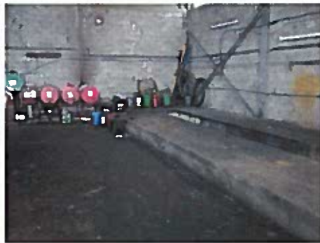
Workshop Bulk and General Cargo – Pit for repairs and oil change
